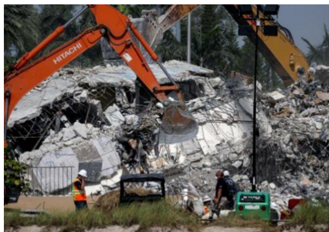
Careful Removal of Building Debris
