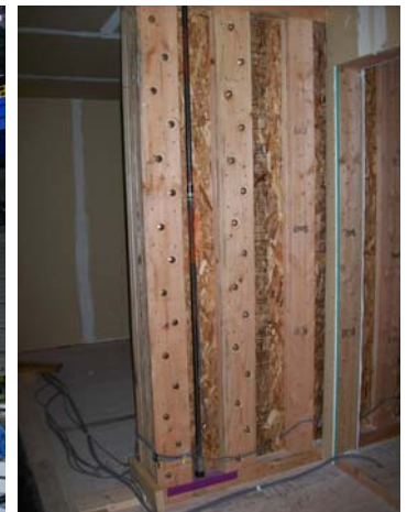
Mid-ply wall in interior
