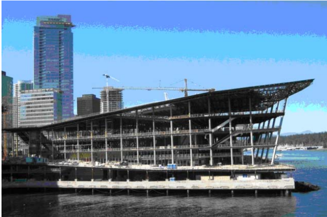
East Elevation Steel Framing
