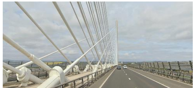
Queensferry's overlapping cable fans viewed from the bridge deck
