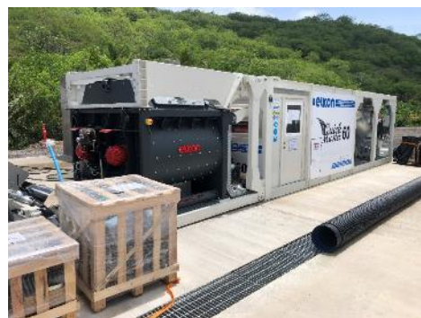
Module batch plant being unpacked and assembled onsite.
