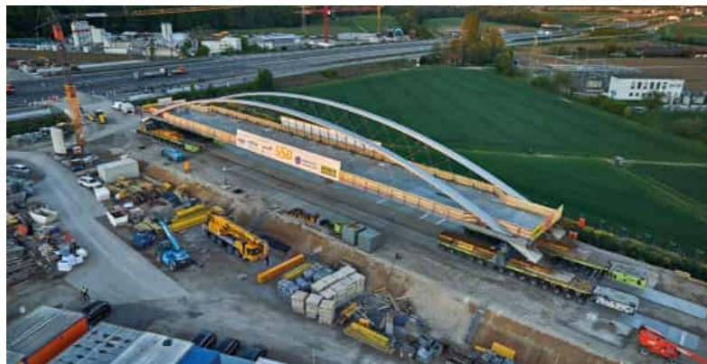
→ Roll-in of network arch bridge
