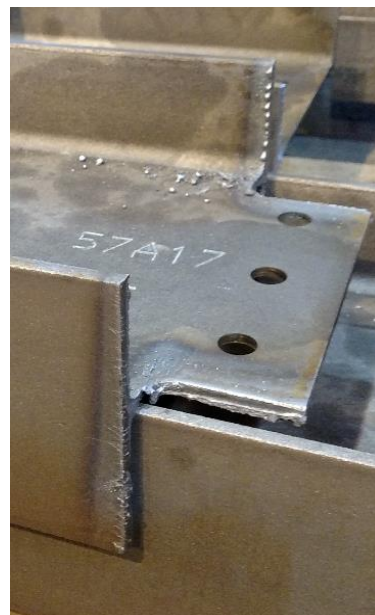
A coped beam- Photo Credit AISC
