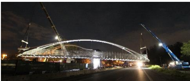
Tynehead Pedestrian Bridge over Highway 1 – Night time erection
