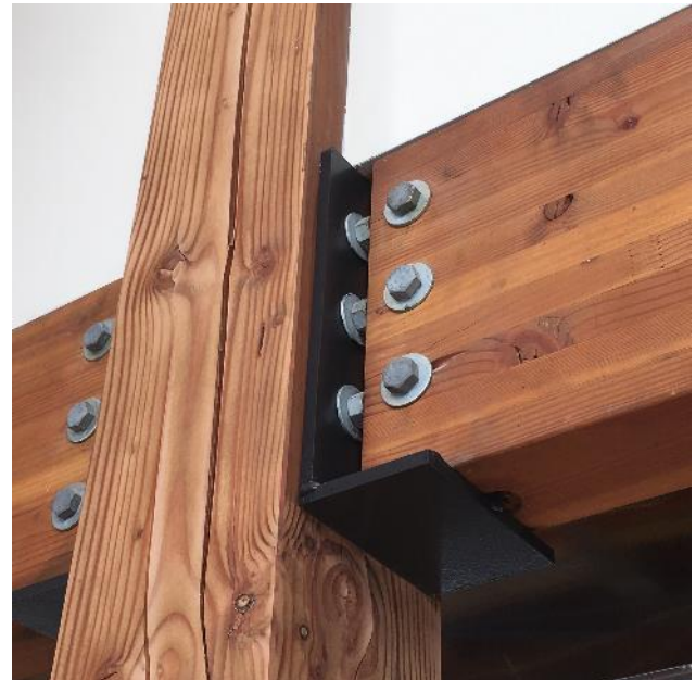
Bolted timber connection at the Vancouver Island Regional Library in Chemainus
