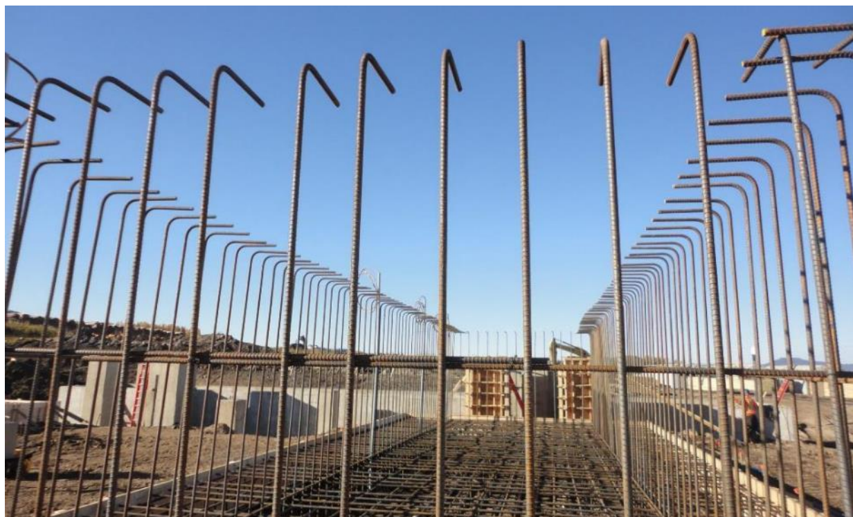
Turbine Inertial Block Foundation, Fraser Lake, BC" by Gairns Santos Engineering Inc.
