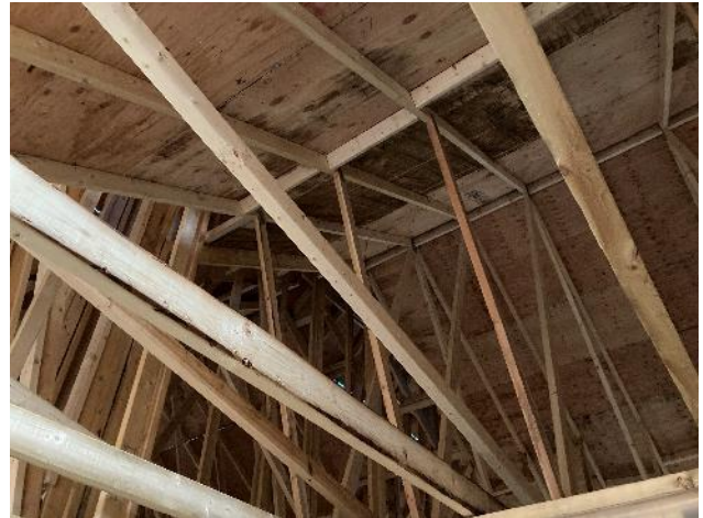
Engineered roof trusses from a rebuild in Mission
