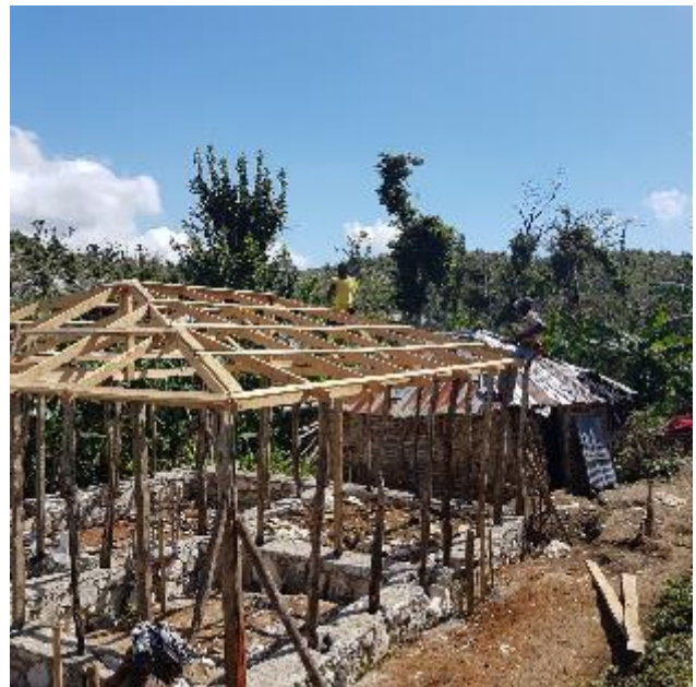
Trained carpenters installing lumber from the kit to rebuild the roof
