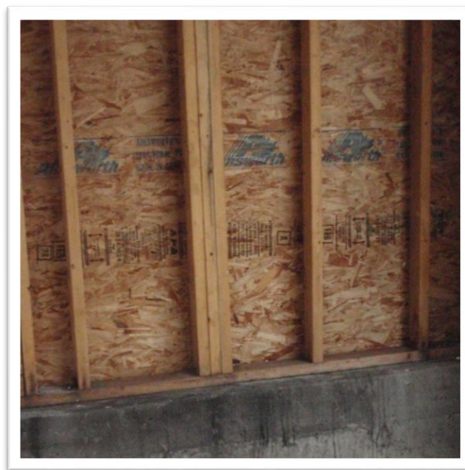
Figure 1: Built-Up Lumber Column in an Exterior Wall
