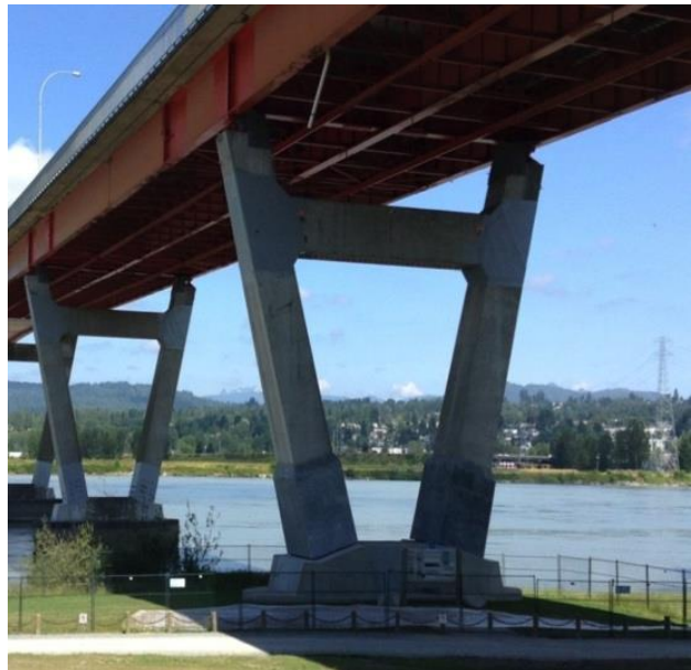
Figure 5: Finished UHPFRC retrofit of Pier S4.
