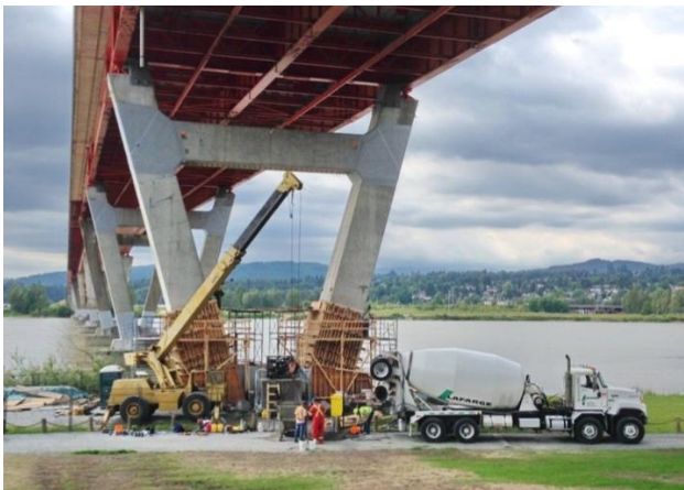
Figure 4: Casting of UHPFRC jacket.
