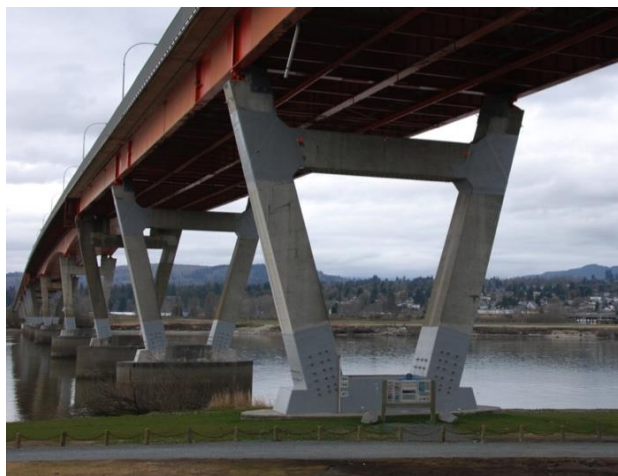
Figure 2: Pier S4 (looking north-east) prior to retrofit with UHPFRC jackets.
