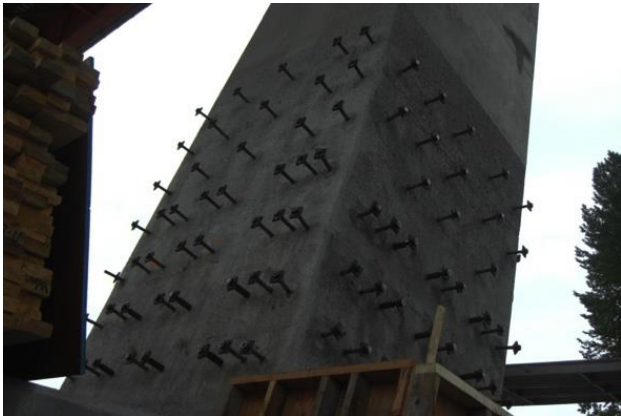
Figure 3: Pier S4: Column preparation with sandblasting and installation of dowels.
