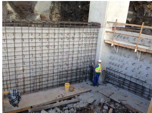
Figure 3: Typical Grade Beam Retrofit
