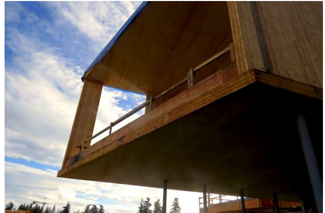
The 4-meter cantilevered dance studio featuring 7ply CLT floor panels to achieve minimal vibration.
