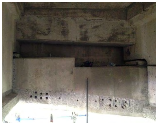
Figure 6: Corbel Dowel Holes for Offset Flange Rebar
