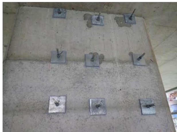
Figure 4: West Pier Column Surface Anchors
