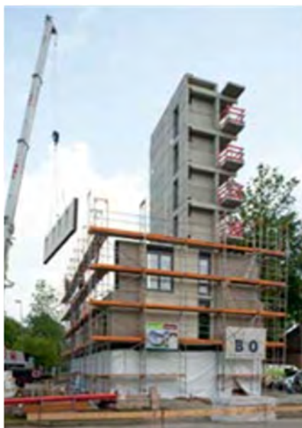
Prefabricated panel installation at Holz 8 Architecture by Schankula Architekten Photo Credit Huber & Sohn
