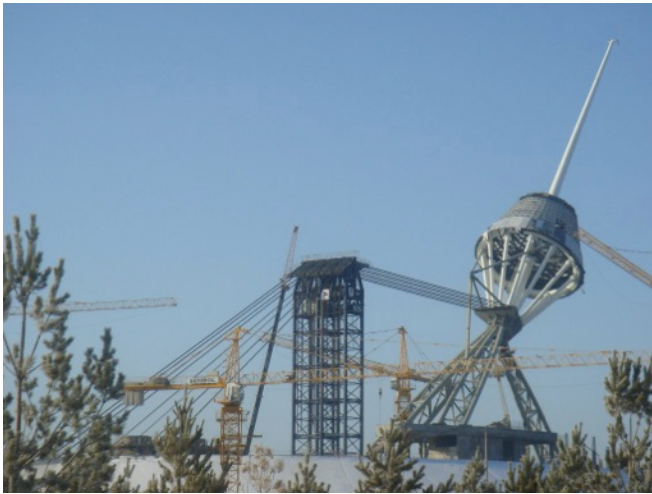
Khan Shatyr Tripod Erection
