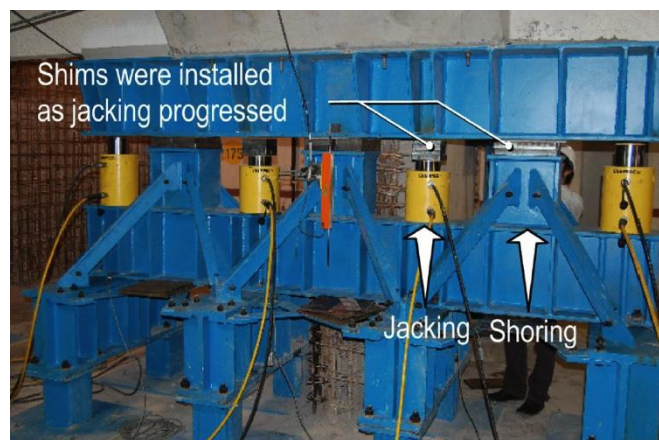
Fig. 6 – Close-up of jacking/shoring system below each wall.
