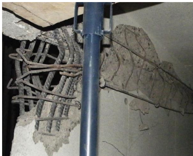
Fig. 2 – Close up of damage in one transverse shear wall.
