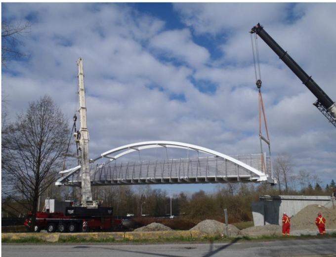
The first Tynehead arch is positioned by two cranes.
