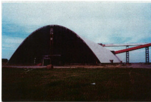
PLATE 14.3 A large potash storage building (70 m clear span) assembled using glulam rivets and prestressed lengthwise to improve lateral stability of the arches.
